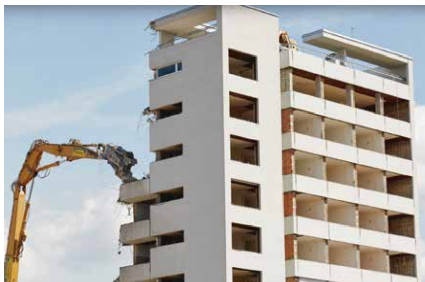
Abbruch Theodosianum April 2015
