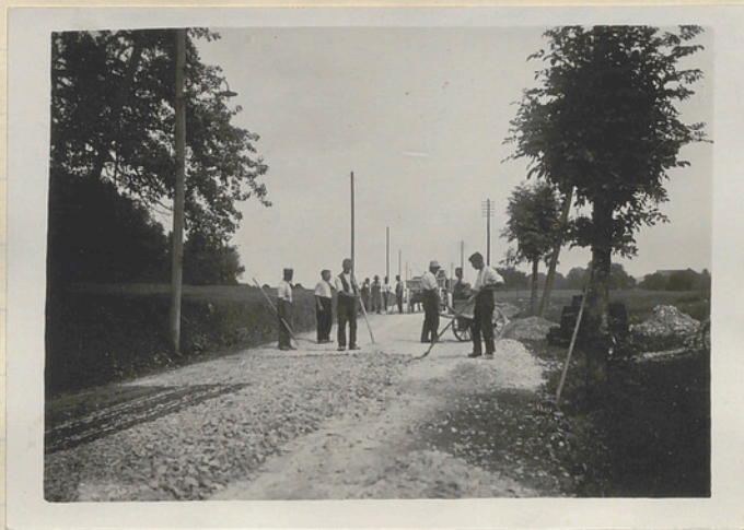
Legen des Schottermaterials Loch-Grimmethall.
